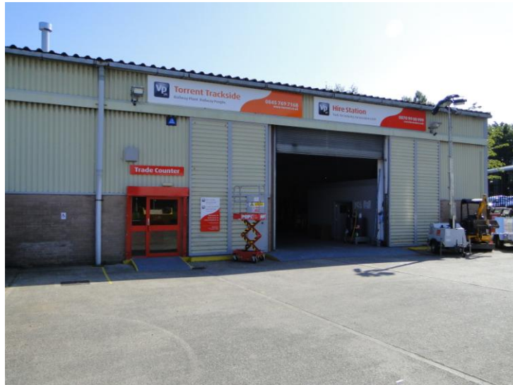
Hire Station Carlisle branch
